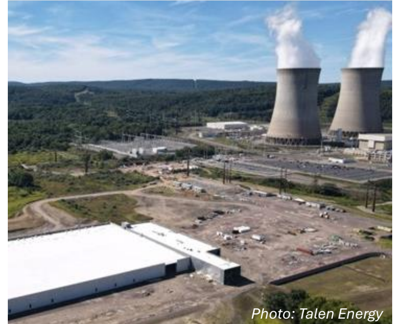
Susquehanna Nuclear Plant and Data Center
