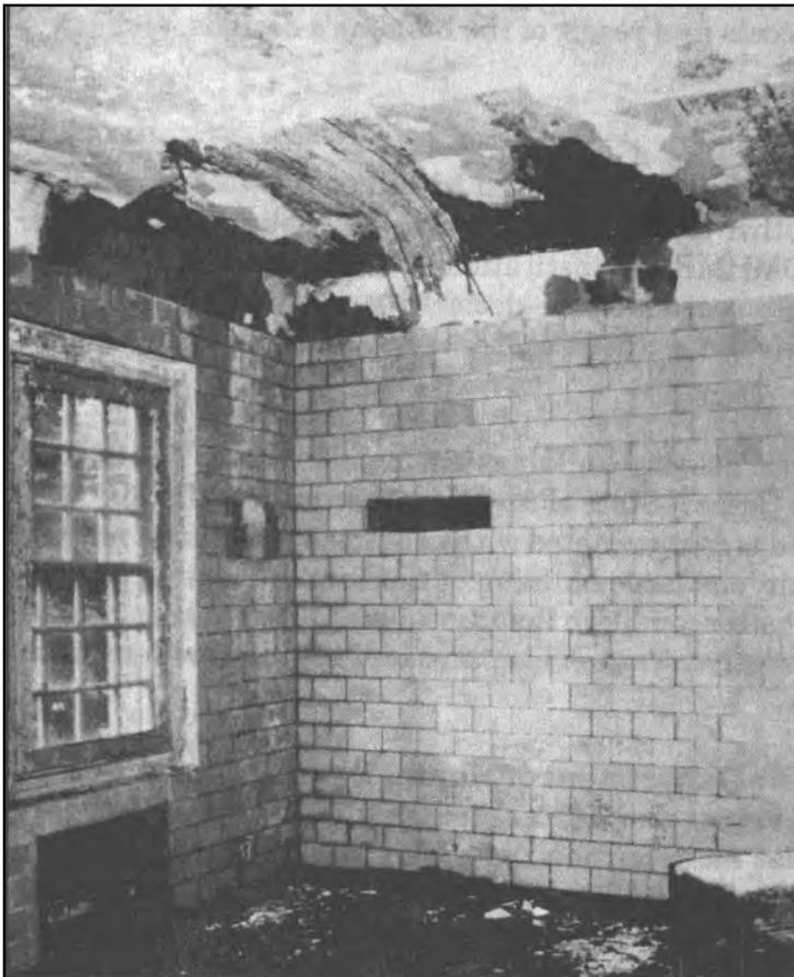
Many mental hospital buildings are in poor repair. The large building at Central State Hospital shown above is severely deteriorated and contaminated with asbestos. The interior view at left shows the extent of the deterioration. Buildings that have fallen to this level of deterioration are probably unusable and unrepairable, and they must be considered liabilities in terms of property value.
